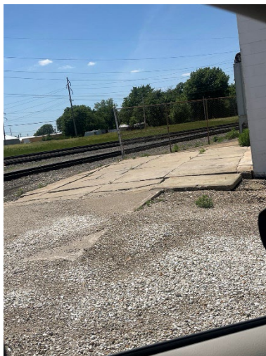
Cracked/broken pavement.
